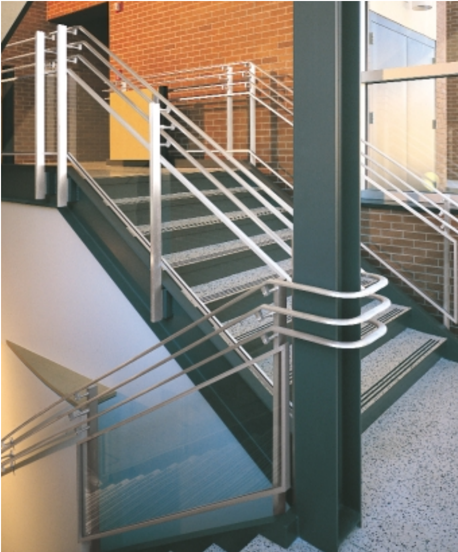
The Fannin Library at Phoenix College, Phoenix, AZ Architect: Durrant Architects Fabricator: Bernie's Brass, Inc., Phoenix, AZ
